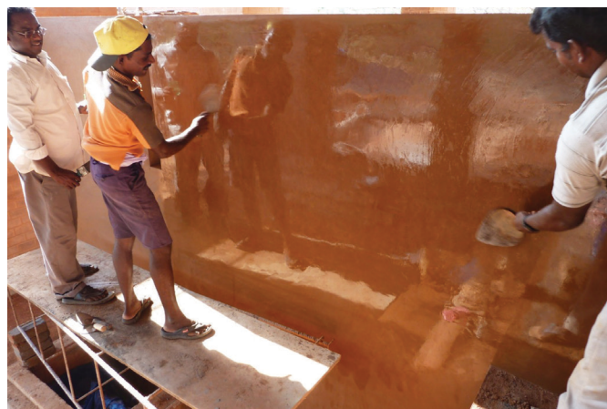
↑ Hand-trowelled mirror finish to earth plastered wall.
