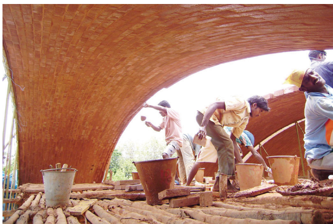
↑ Free-spanning optimised vault built without formwork.
