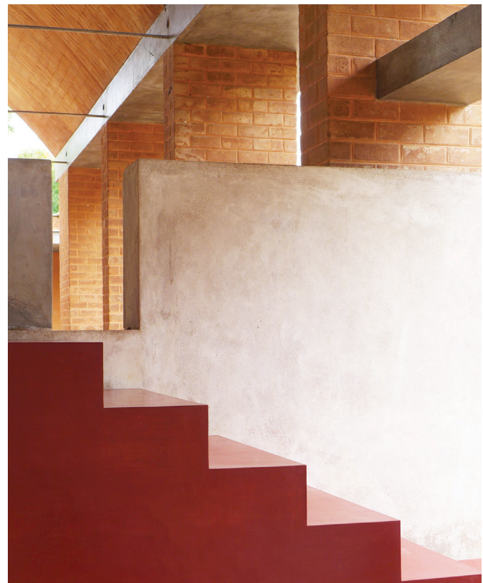
↑ Materials Detail: Natural pigments, lime plaster, polished concrete, earth blocks.
